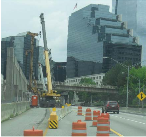
Lane closures and barrier removal in preparation for installation of footings for MARTA Bridge project.
